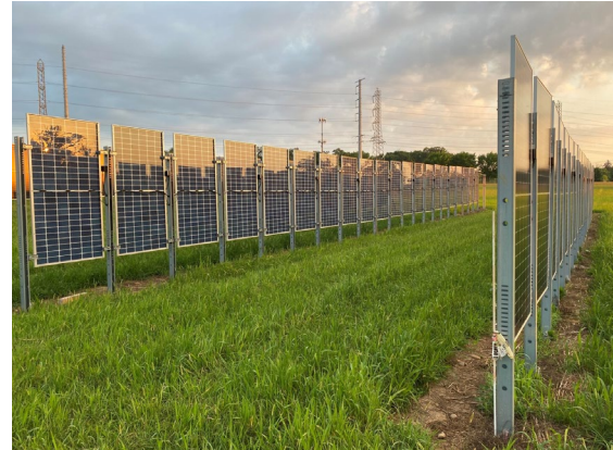
Figure 3: Vertical bifacial array, looking North, at the Rutgers University Animal Farm on Cook Campus, New Brunswick, NJ. Image © Rutgers Agrivoltaics Program.
