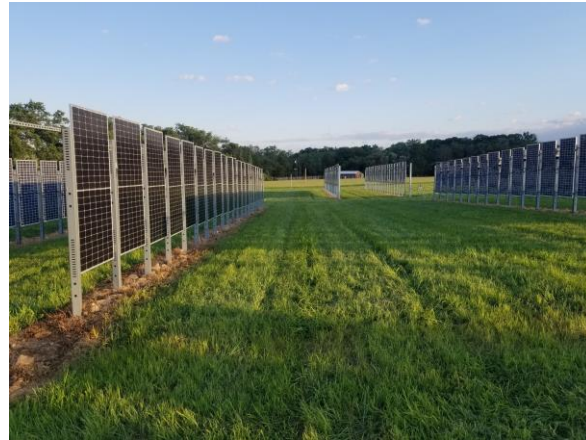
Figure 3: Vertical bifacial array, looking South, at the Rutgers University Animal Farm on Cook Campus, New Brunswick, NJ.
