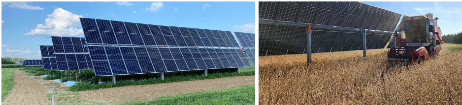
Crops are grown underneath and adjacent to tracking solar arrays. Module tracking movement can be altered for a time period to improve seed germination and early plant establishment.
