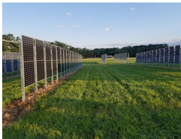
Figure 3: Vertical bifacial array, looking South, at the Rutgers University Animal Farm on Cook Campus, New Brunswick, NJ.
