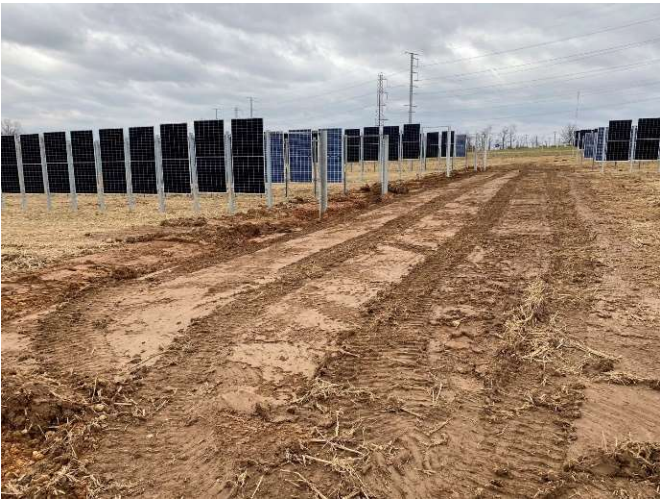
Soil compaction
