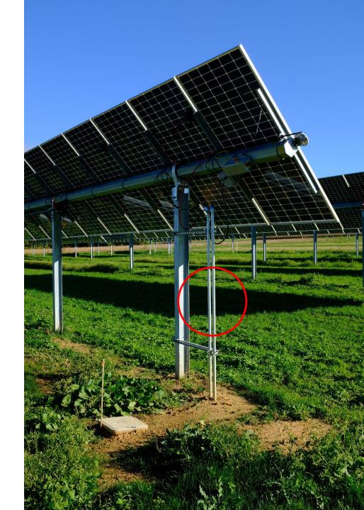
Incorrect placement of in-ground conduit boxes: Obstruction for jarming equipment
