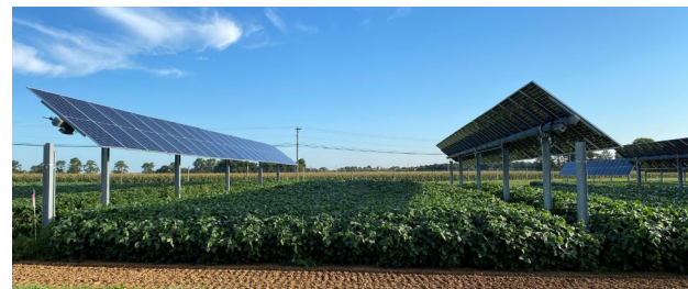
Figure 2: Single-axis tracking array, looking North, at the Rutgers Agricultural Research and Extension Center, Bridgeton, NJ.
