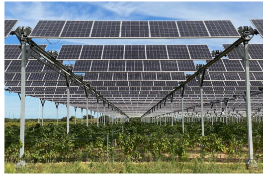
Figure 1: Examples of agrivoltaic installations. Top left: single-axis trackers with a single row of panels; top right: single-axis trackers with a double row of panels; bottom left: vertical bifacial panels; bottom right: elevated single-axis trackers. Image credits: Top left, top right, bottom left: Rutgers Agrivoltaics Program, bottom right: https://www.reuters.com/ (no endorsement implied).
